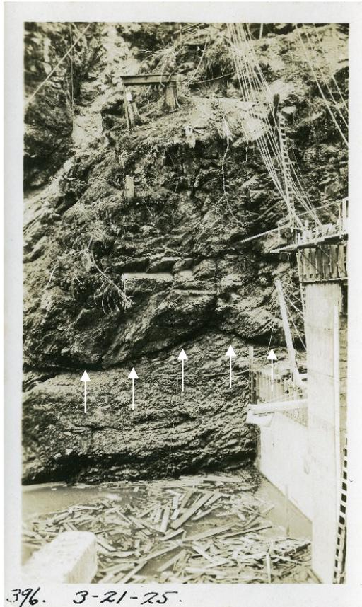
Figure 6. Example of construction photo from 1925 showing the bedrock immediately upstream of the dam in the left abutment in what is now the reservoir. Note the presence of an irregular sub-horizontal fault in the centre of the image (white arrows).
