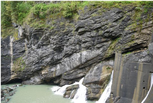
Figure 2. Leakage along structural pathways in the bedrock of the right abutment.
