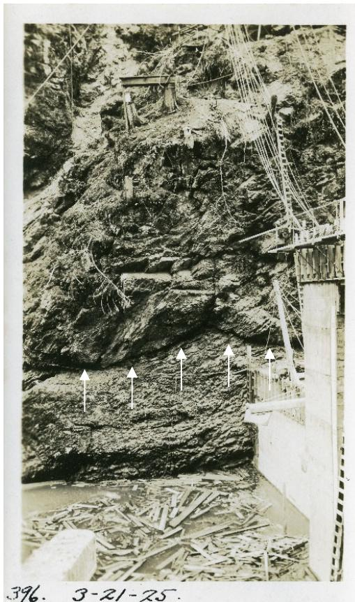
Figure 6. Example of construction photo from 1925 showing the bedrock immediately upstream of the dam in the left abutment in what is now the reservoir. Note the presence of an irregular sub-horizontal fault in the centre of the image (white arrows).
